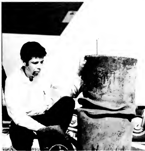
Photo 51. Compressive forces buckled 16" steel gas pipe in Glonaaks Boulevard, San Fernando. Southern California Gas Co. photo.
